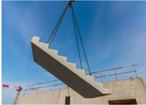
PREFABRICATION (STAIRS & FLOORING)
