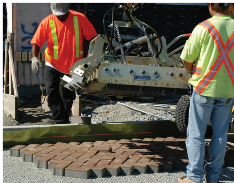
Fig. 3.42—A unique 45-degree herringbone paving pattern eliminated removal and replacement of half-stones, thereby saving labor expense and reducing paving time. The layers arrived at the site in a 45-degree pattern with no shift or misalignment during transport. Photo courtesy of Interlocking Concrete Pavement Institute
