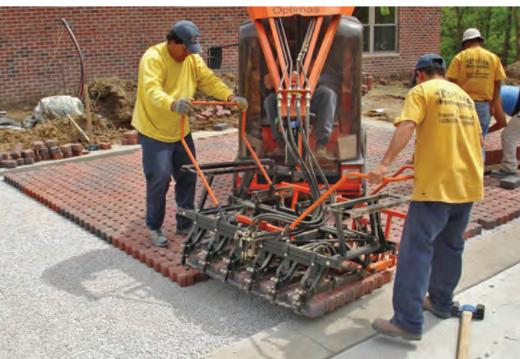
Fig. 3.34—Mechanical installation equipment places ready-made layers of the concrete pavers. Photo courtesy of Interlocking Concrete Pavement Institute
