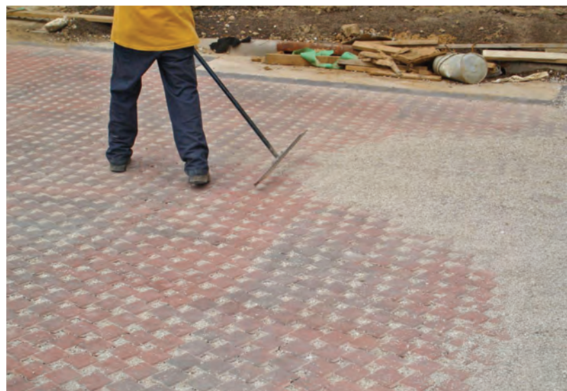
Fig. 3.36—The paver openings are filled with the small stones (CA-16), and excess stones are removed from the paver surface before compaction. Photo courtesy of Interlocking Concrete Pavement Institute
