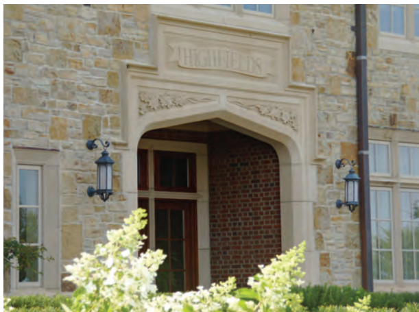
Fig. 3.17—This private residence incorporated a large amount of cast stone, which included a custom designed ornate entry, window surrounds, water table, clad columns, roof coping, and site wall coping (Lewisburg Residence, PA). Photo courtesy of Cast Stone Institute
