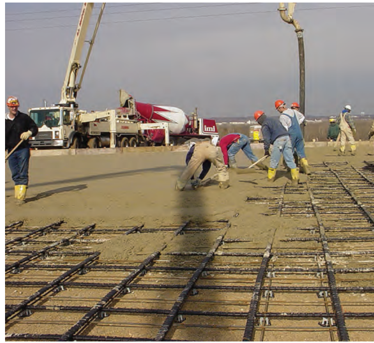
Fig. 3.23—Placing a cast-in-place post-tensioned foundation.
