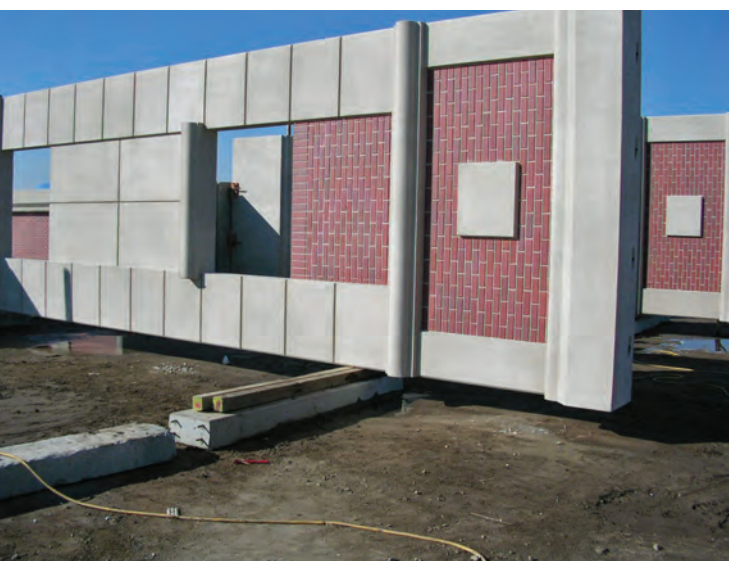
Fig. 3.7—The completed architectural precast panel with all the components included window sills, quoins, and coping. Photo courtesy of National Precast Concrete Association
