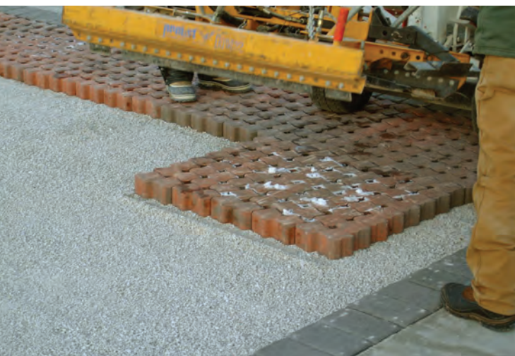
Fig. 3.33—The permeable interlocking concrete pavers are supplied and installed in layers on the screeded bedding material (pea-sized aggregate—bedding sand is never used in PICP). Note the snow on the pavers doesn't interfere with installation, and the border coarse against the concrete curb provides a finished edge. Photo courtesy of Interlocking Concrete Pavement Institute
