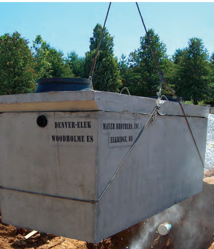
Fig. 3.65—Precast grease interceptor. Photo courtesy of National Precast Concrete Association
