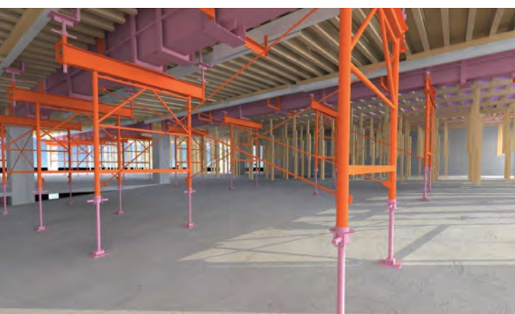
Fig. 2.4—Rendering of suspended slab formwork systems used during construction. Rendering courtesy of Virtual Design & Construction Dept., KLORMAN Construction
