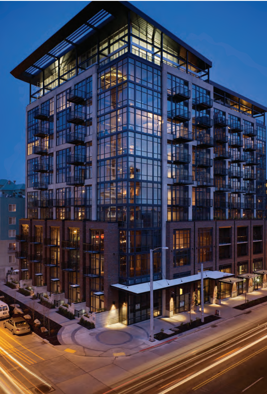
Fig 3.16—Cast-in-place concrete frame with post-tensioned flat-plate slabs are used in construction of the Mosler Lofts in Seattle, WA. Photo courtesy of Post-Tensioning Institute
