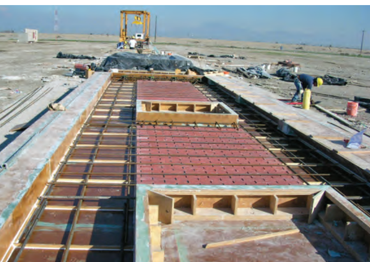
Fig. 3.6—Precast form with thin brick installed in a form. Photo courtesy of National Precast Concrete Association
