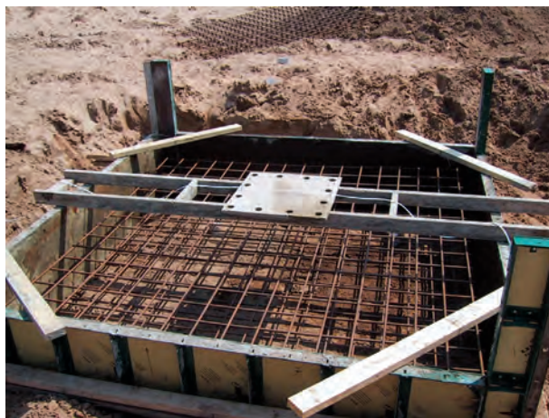
Fig. 1.24—Welded wire reinforcement placement in footing (Ice Mountain). Photo courtesy of ACI Committee 439 volunteers
