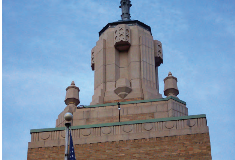
Fig. 3.21—Restoration (before and after): cast stone was used to replicate the entire original exposed aggregate structure, while maintaining the historical integrity of the intricate architectural details (Naples Central School District Naples, NY). Photo courtesy of Cast Stone Institute
