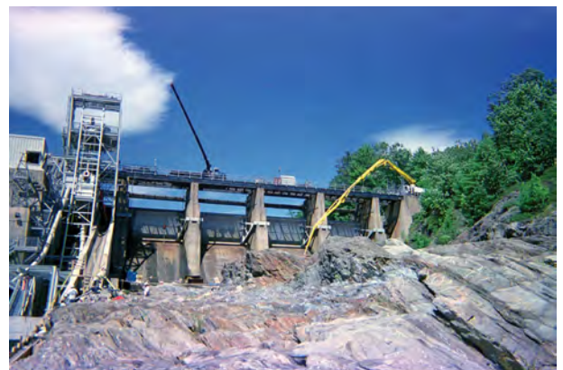
Fig. 2.24—To reach the furthest point of concrete placement, Northeast Concrete Pumping positioned their boom pump on land's edge, then fully extended the 151 ft (46 m) long boom to the ground below and finally connected the pump's end hose to 340 ft (104 m) of four-inch delivery system. Photo courtesy of Putzmeister
