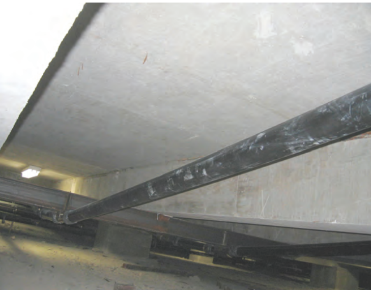
Fig. 4.6—External post-tensioning for strengthening concrete beams. Photo courtesy of VStructural, LLC (VSL)
