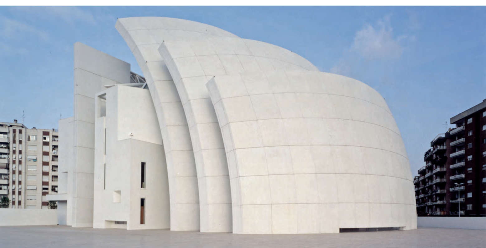
Fig. 1.29—Photocatalytic concrete was used at the Dives en Misericordia Church in Rome, Italy. Photo courtesy of Essroc Cement Corp.
