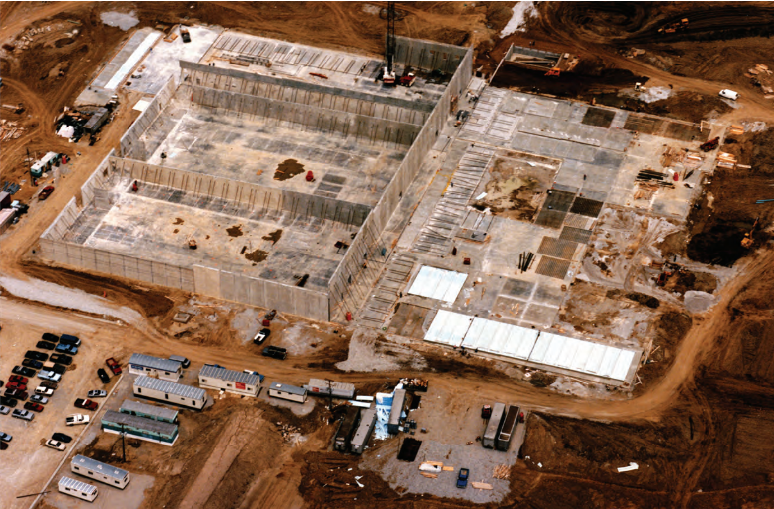
Fig. 3.81—Construction site with tilt-up panels during casting and erection. Photo courtesy of Tilt-Up Concrete Association
