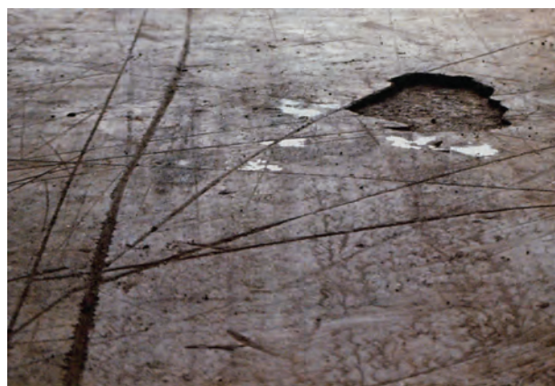
Fig. 1.13—Transfer floor wear after 1 to 3 years. Photo courtesy of Silica Fume Association
