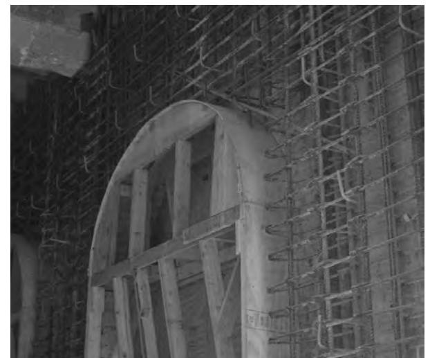
Fig. 4.19—Interior wall in preparation for shotcrete application. Photo courtesy of American Shotcrete Association
