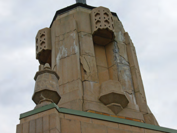
Fig. 3.21—Restoration (before and after): cast stone was used to replicate the entire original exposed aggregate structure, while maintaining the historical integrity of the intricate architectural details (Naples Central School District Naples, NY). Photo courtesy of Cast Stone Institute
